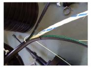
Unwrap fiber tubes and remove strength member leaving 3"to secure to hardware at the next step.
