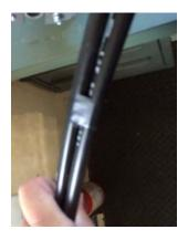
Once that is complete then measure between 8' to 9' from the ends and put a ring cut (for a D closure) and approximately 6' for a B enclosure.
