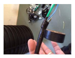
Choose the best length of strength member hardware and install onto the cable securing with the ring clamp provided.
