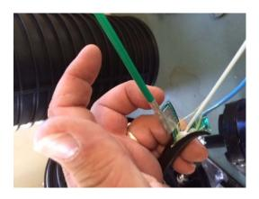
Using black tape wrap it around the grounding hardware and continue to wrap around the cable so that the hardware has something to grip when installing the rest of the hardware.
